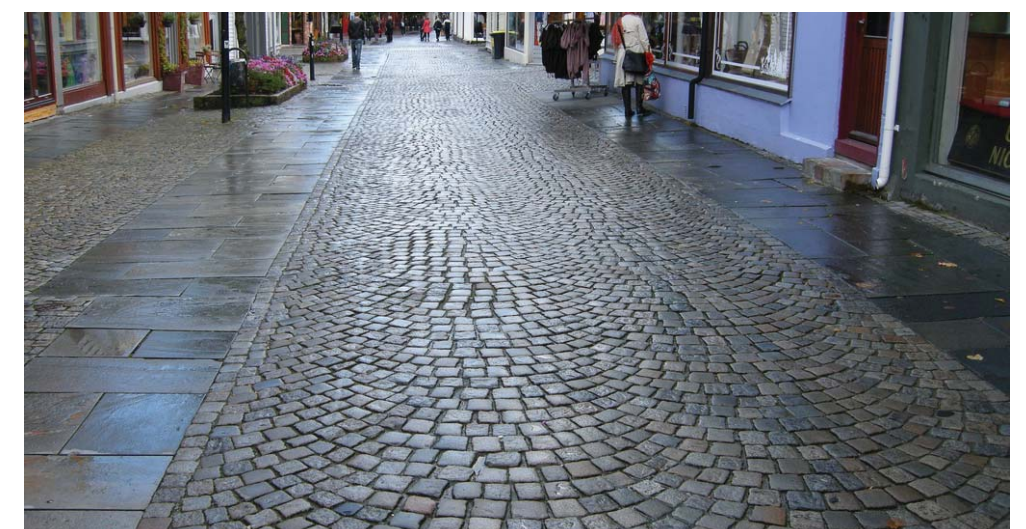
Curbless Paving and Vehicular Overlapping Paving
